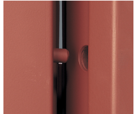
Three fixed bolts in the rear edge.
