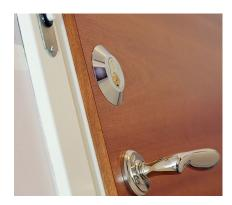
At the main lock, the door leaf has integrated drilling protection.
